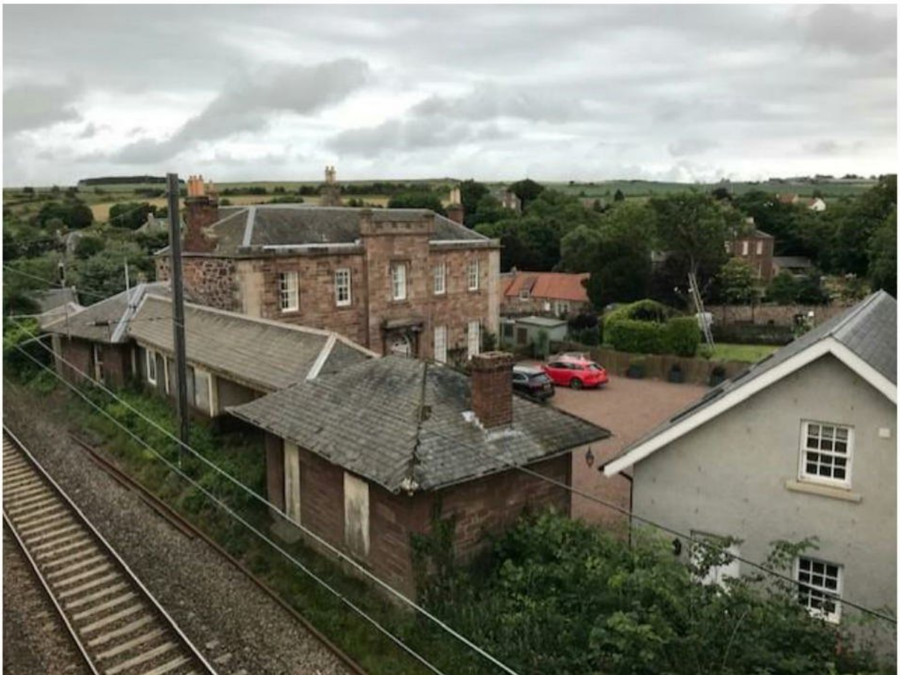
Figure 2 Original East Linton Station (private dwelling)
