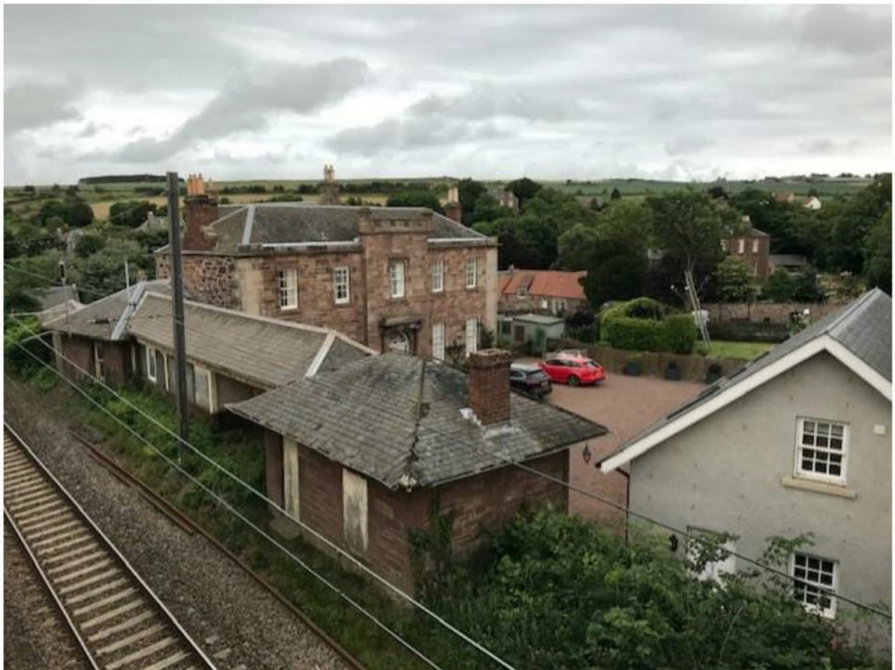
Figure 2 Original East Linton Station (private dwelling)
